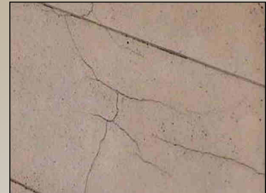
Detail of fissures in stucco
