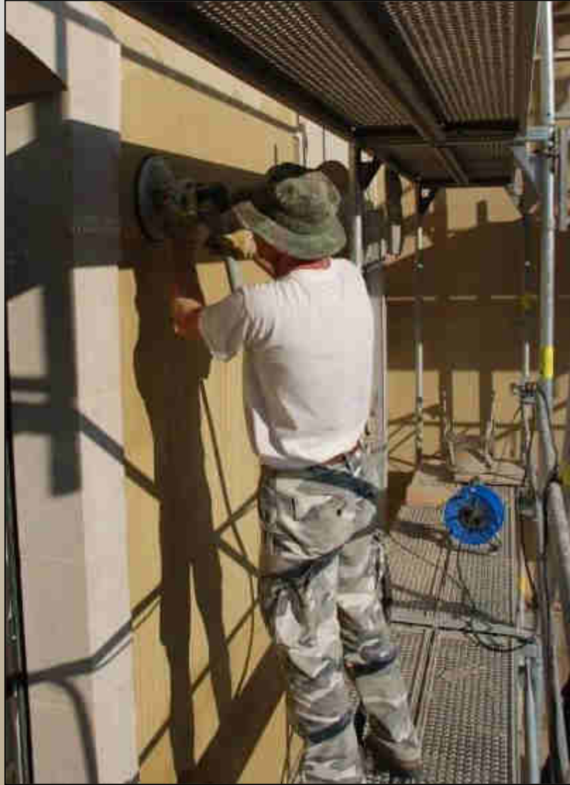
„Planing“ of stucco by Vertika hydraulic grinding machine
