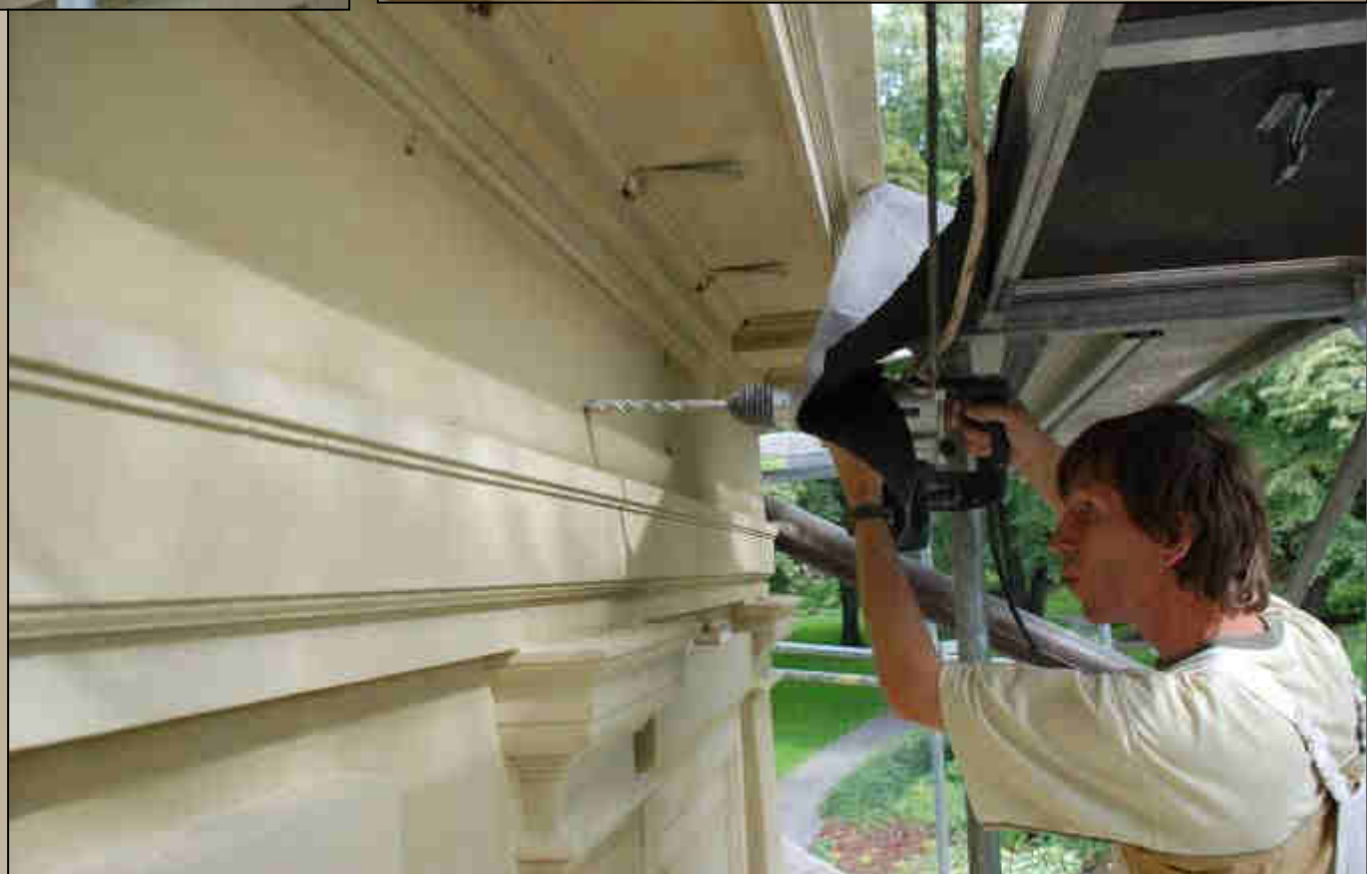
Assembling cast elements on facade
