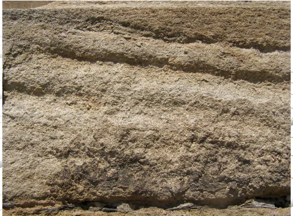
Test 2 : stone ashlar with weathered sedimentary layers
