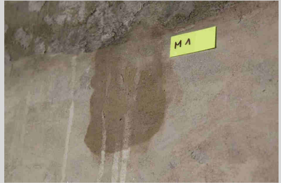
Application of cleaning poultices in Arbocel
