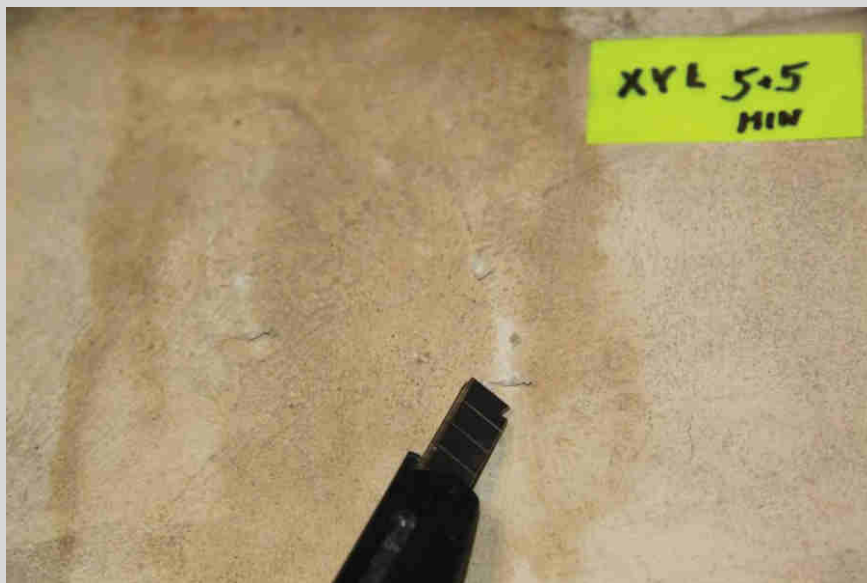
Application of cleaning poultices in Arbocel
